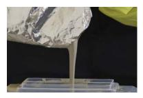
8. Pour pouch contents into the joint shell.
