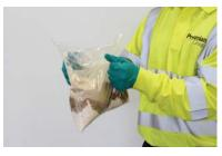
5. Make sure that the membrane seal is completely open before mixing the powder and liquid together.
