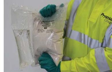
2. Aerate the powder by gripping the pouch at each end and tumbling the powder for up to thirty seconds, this will facilitate mixing
