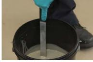
7. Commence mixing with paddle. Add the remaining sand and mix until all sand is wet out.
