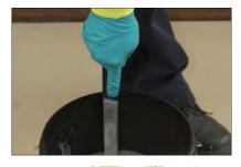
Prysmian low density three part resin has enhanced performance characteristics compared with conventional three part systems. The resin is supplied as a combination of twin pack pouch and supplementary sand filler. Bulk filling with sand allows up to 8 litres to be supplied in a single kit.
