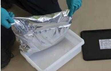
1. Open container and remove foil resin pack. Check bag for any signs of damage before proceeding.
