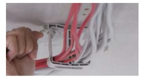
The SH holder forms a closed ring around the shethed cables and can be re-opened using a handle.
